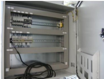
IC 2IN + 1 OUT 7.2kV – 630A 3p outside and inside view of separate control cabinet
